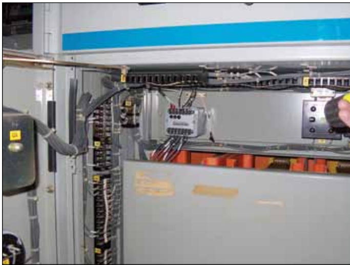
Figure 1 — Transducer Wiring
