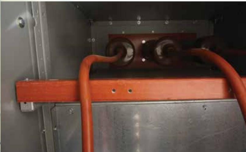
**Figure 5:** *Improper Cable Installation*
