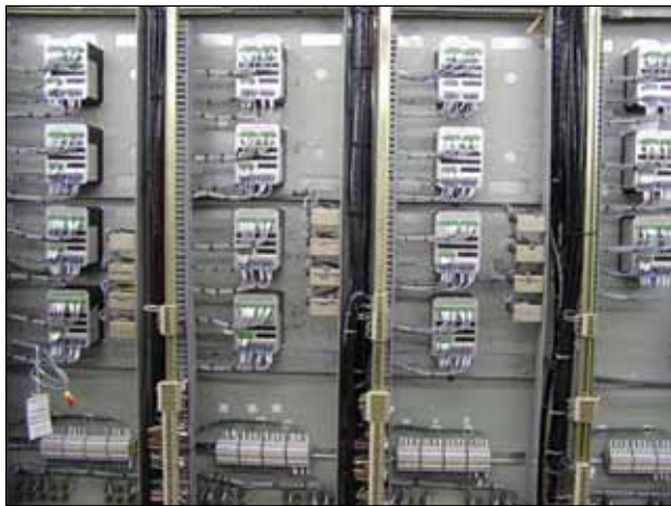
Figure 2 — Motor Protection Retrofit
